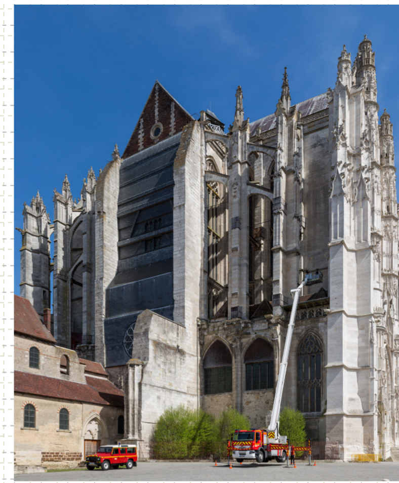
Figure 22: Beauvais Cathedral undergoing refurbishment
