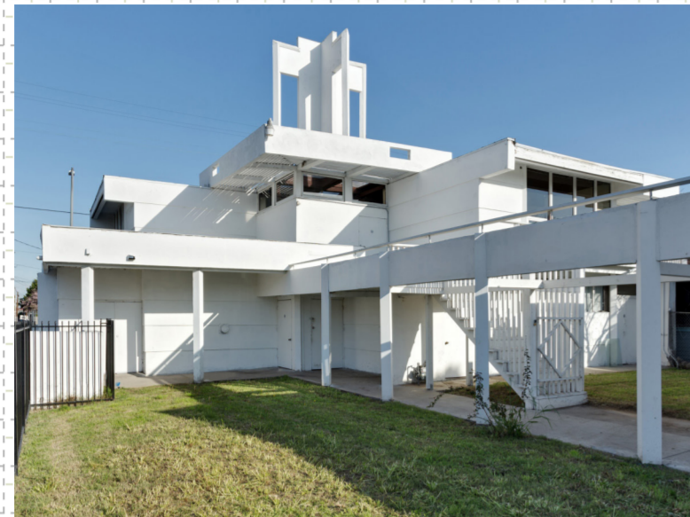
Figure 12: Bethlehem Baptist Church exterior
