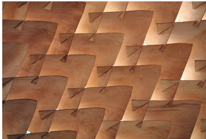
PAVILLION PANEL DESIGN, + ADHESIVE FREE INTERLOCKING
